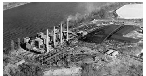
Louisville Gas and Electric Company, Paddy's Run plant, west Louisville, 1949. UNIVERSITY OF LOUISVILLE PHOTO ARCHIVES
